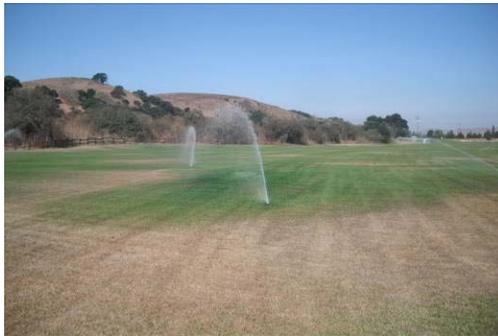
**Dry Spots due to Lack of Coverage & Clogged Rotors Not Rotating**
